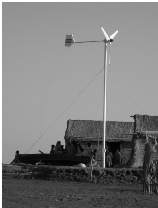
Figure 8: Use of Alternative Energy - Wind Turbine
